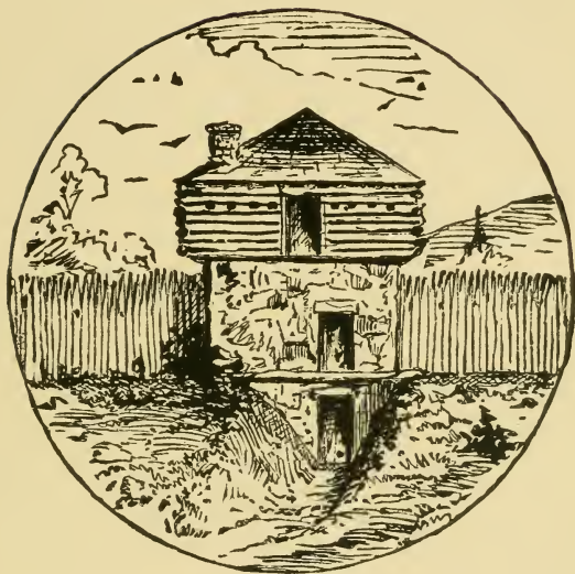
Block House, Built in 1780.
